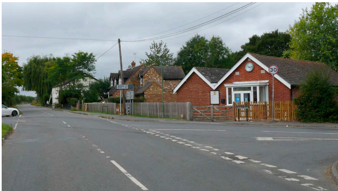
Braywood Memorial Hall
